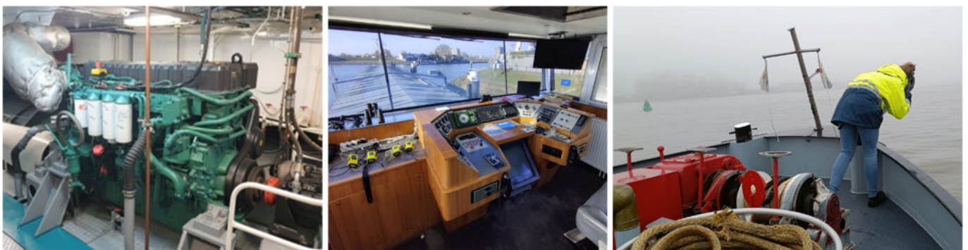
Left: Engine Room
